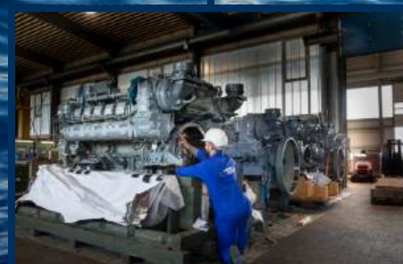
Main and auxiliary engine works
